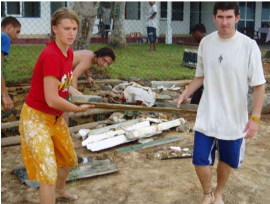
Volunteers carrying the debris to the trailer
